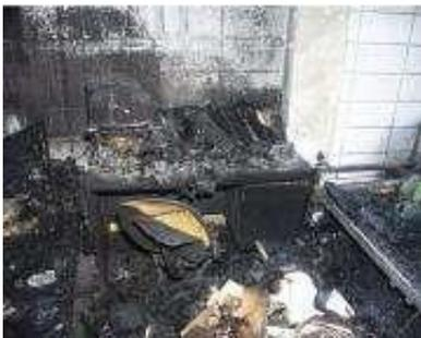
These post-fire photographs of the dorm rooms show the difference a sprinkler makes. There is little visible damage in the top photo that had a sprinkler in the room; there was no sprinkler in the dorm room in the lower picture. Credit: NIST
